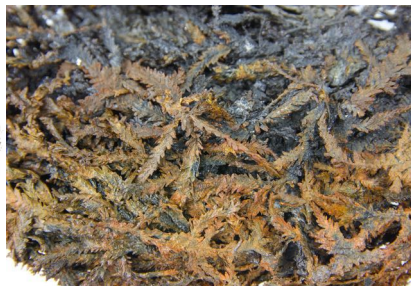
moss caulking in scarf
